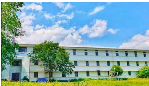
Fig – RCC Boys Hostel
