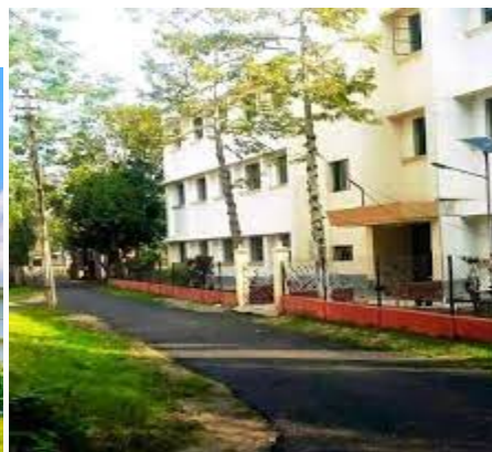
Fig- RCC Girls Hostel
