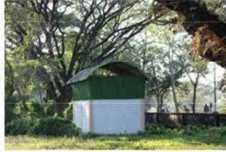
Incinerator in the GU Campus
