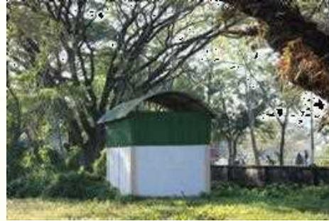
Incinerator in the GU Campus
