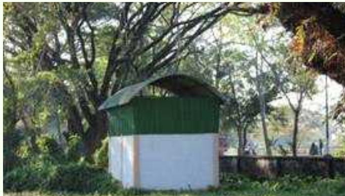
Incinerator in the GU Campus
